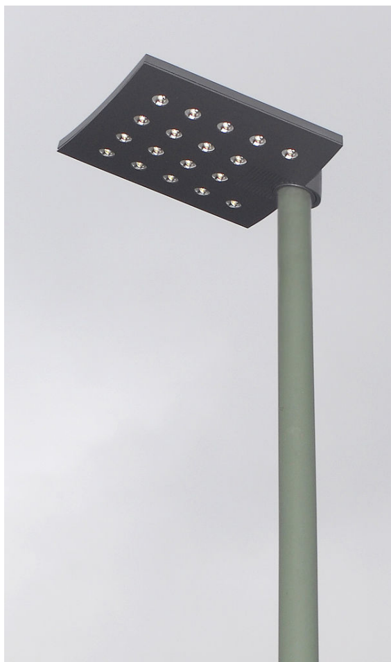
Street light combining a solar cell power source with LED lamps and supercapacitors for energy storage
